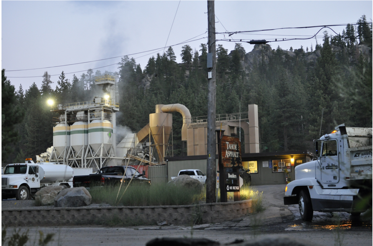
Tahoe Asphalt plant has been operating in South Lake Tahoe for more than 50 years. Photo/Provided
