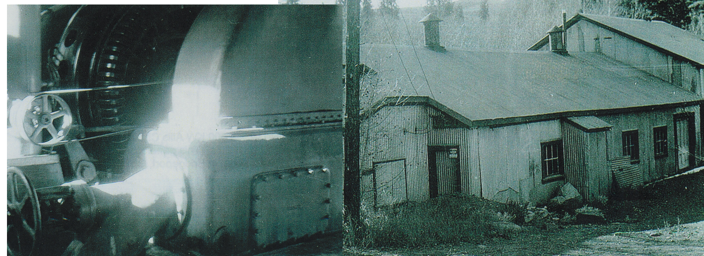
Green Creek Generator
